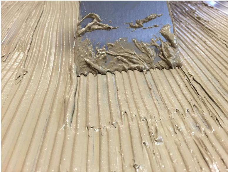
Thermal mastic must be spread with a grooved trowel for even an even coating on the underside of the granite.
